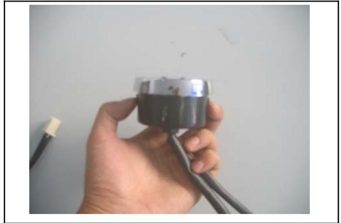
c. Install new meter and press down in to the meter casing.
