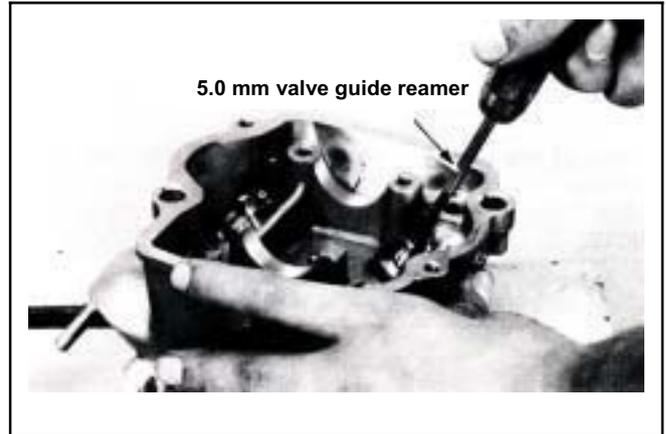
Measure and record each valve guide inner diameters.
